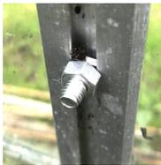
Fix a cropped head bolt with a nut into the slot of the greenhouse frame at each mark, leaving the bolt thread exposed; you'll fix the P-clips to these. Some greenhouses have slightly larger slots, which do not lock the cropped head bolt, but you will still be able to tighten the nut up with care.
